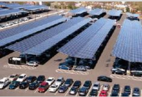
Commercial car park
